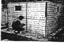
Photo 4. Specimen During Construction
